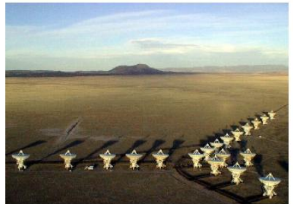
Figures 69 The "Very Large Array" (VLA) of radio telescopes. The twenty seven telescopes can be spread out to a diameter of 36 kilometers.
