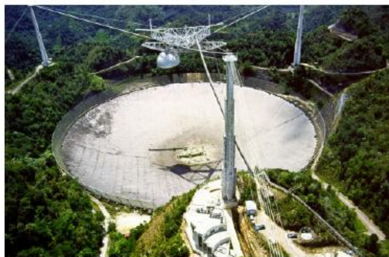
Figure 68 Arecibo radio telescope. While the world's largest telescope dish remains fixed in the earth, the focal point can be moved to track a star.
